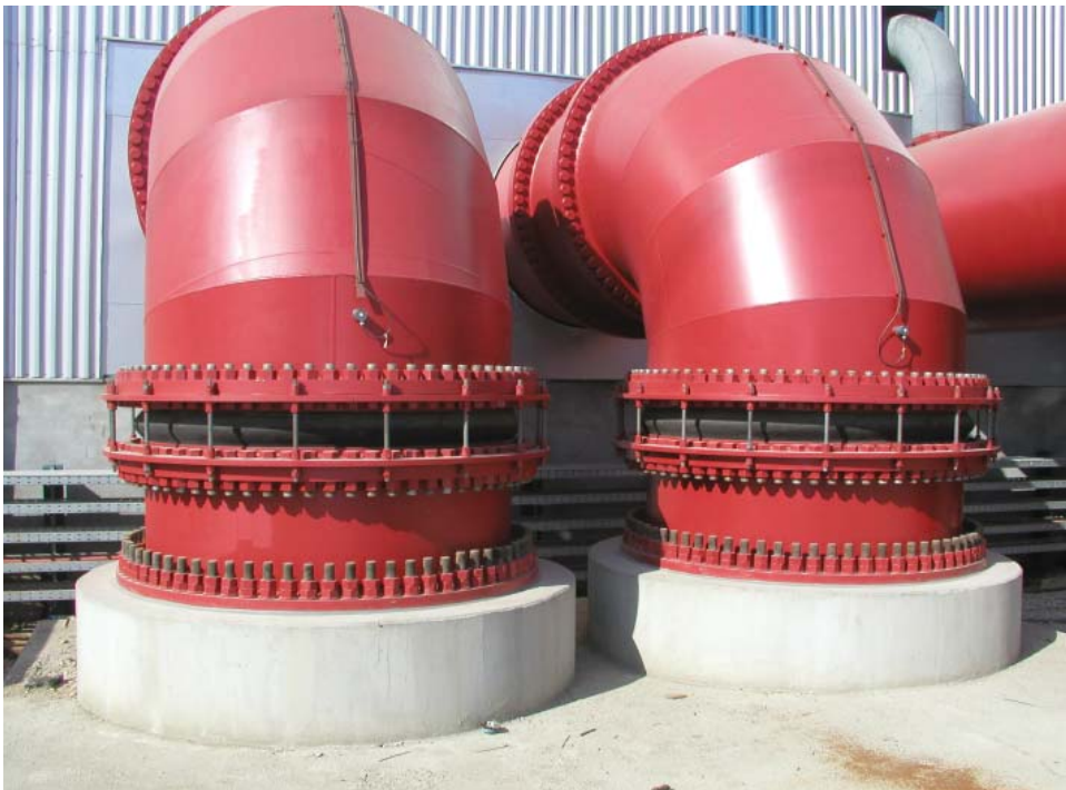
restraint compensator - design M DN 2600
