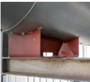
Lift-off restraint
