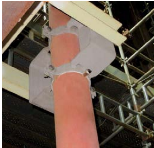
Pipe bearing (type 49 ... -G2P)
